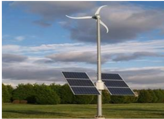
Figure 1. Installation of solar panels with a wind turbine.
