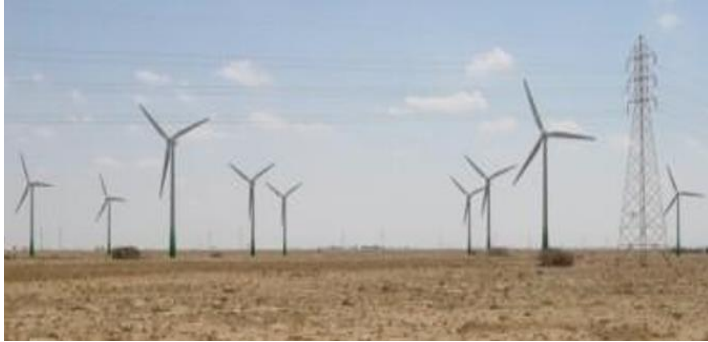
Fig (3) Wind farm in Darnah
